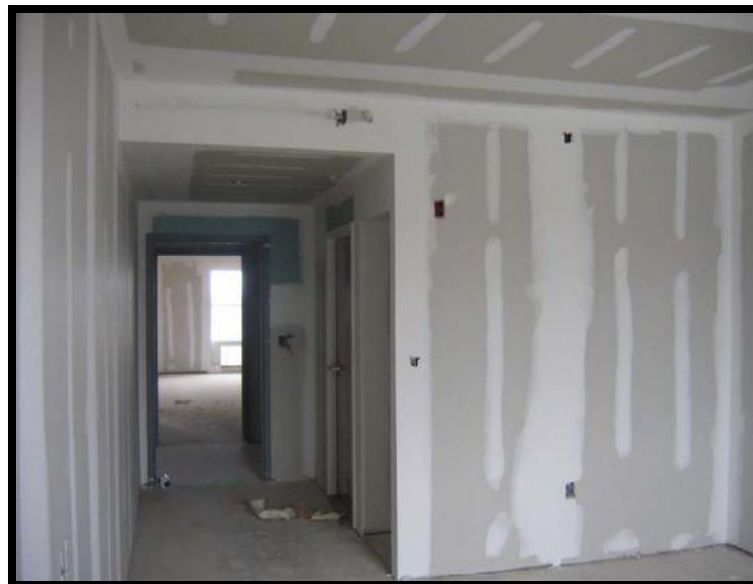
Figure 44: Framing the Pods into the Building (Mensh)
