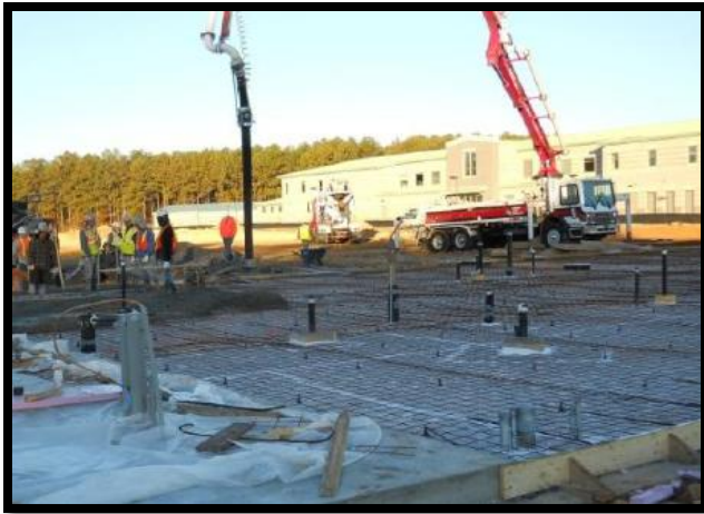
Figure 14: Slab on Grade - Courtesy of Barton Malow
