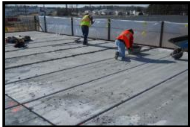
Figure 15: Hollow-core Planks - Courtesy of Barton Malow
