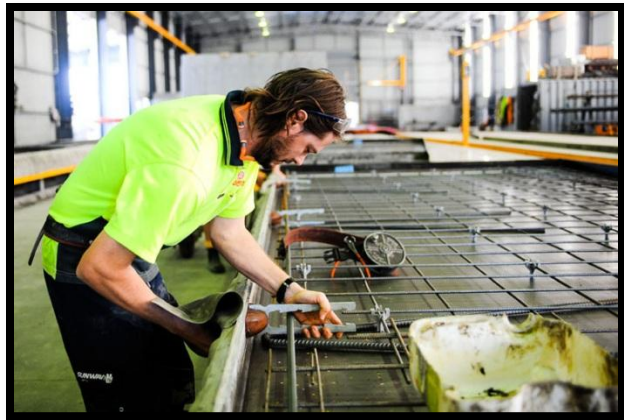
Figure 87: Repetitive Practices (“Gate Precast”)
