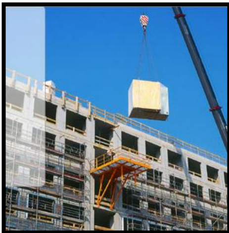
Figure 36: Placement with Crane (Mensch)
