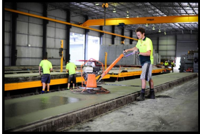
Figure 89: Working Environment (“Gate Precast”)
