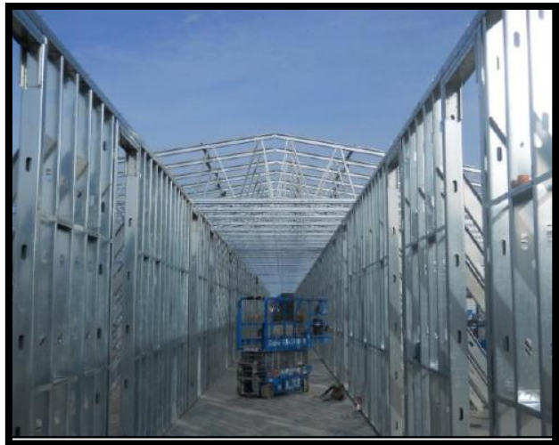
Figure 13: Metal Stud Bearing Walls - Courtesy of Barton Malow
