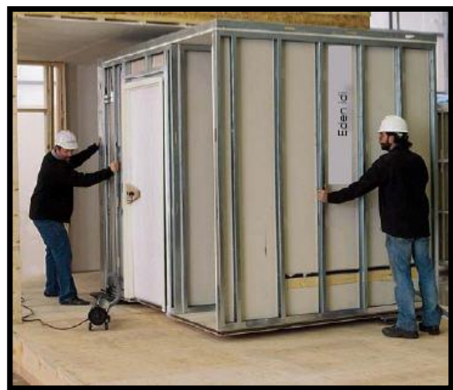
Figure 41: Moving Pods into Place (Mensch)
