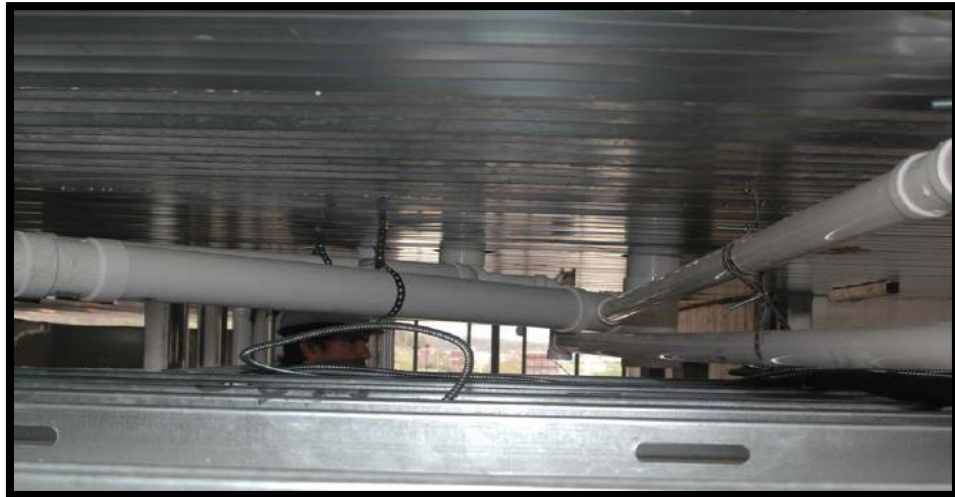
Figure 43: Plumbing Hookups (Mensh)
