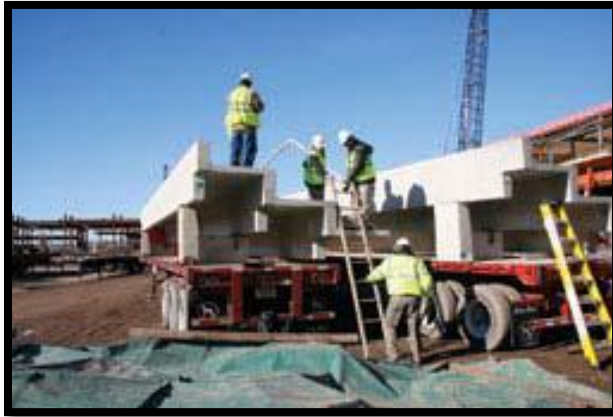
Figure 101: Precast Members Being Delivered - (Sawyer)
