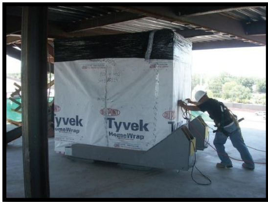
Figure 37: Pod Being Moved into Temporary Locations
